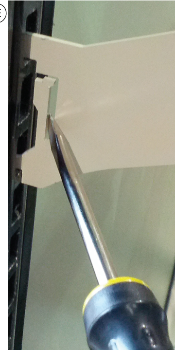
INSTALL CENTER DIVIDER BRACKET
